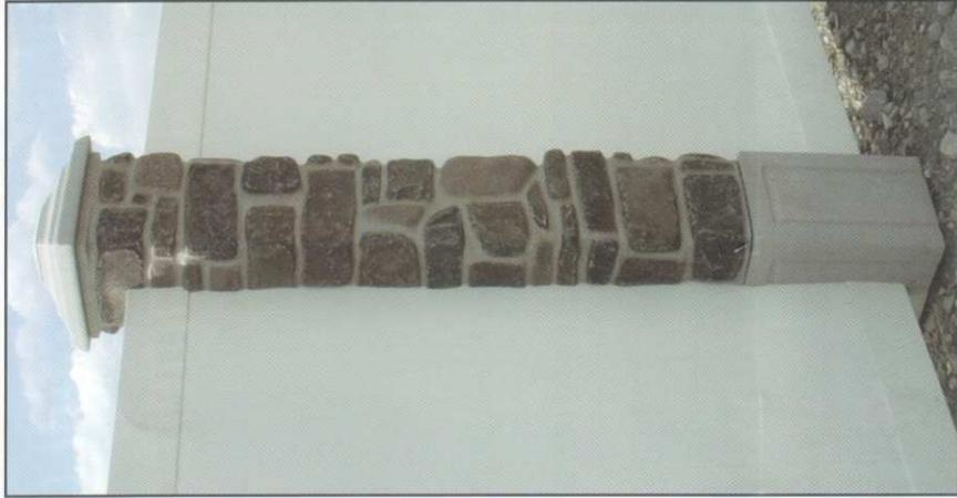
Six foot privacy fence with Reproduction Rock Post installed on top of riser.
